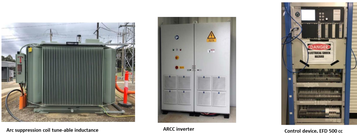
Figure 5: Three components to ARCC technology
