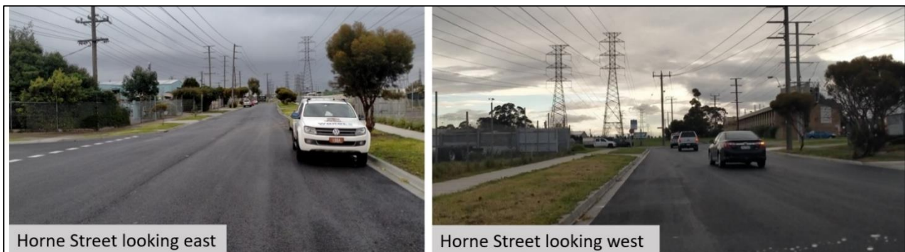
Figure 2-5: Horne Street Site Visit Photos
